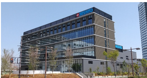
R&D International Exchange Center Building A
